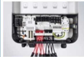
Inverter and transformers
