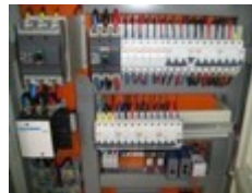
Electric Management System
