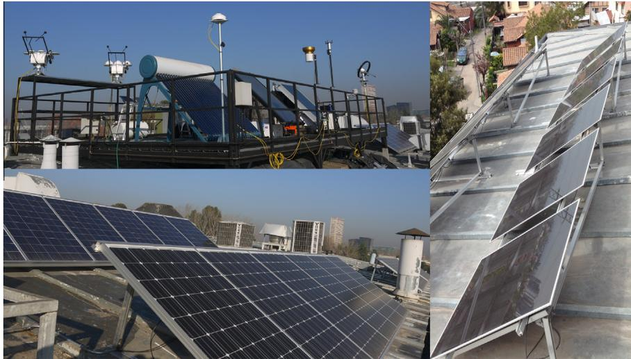
Fig. 1. PV Plant showing climate sensors and PV arrays of mono-, polycrystalline and thin films solar panels.
